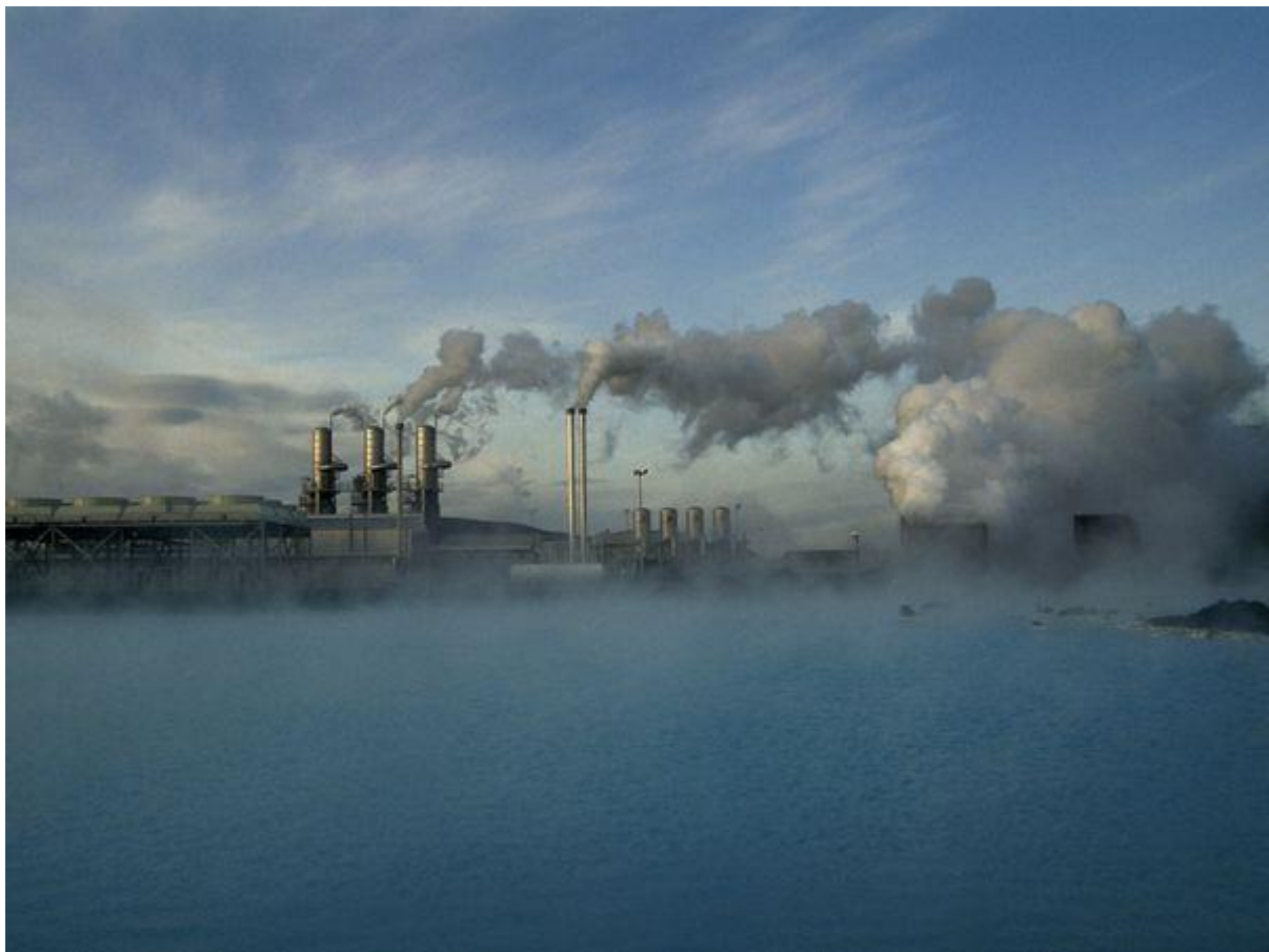
(Medford Taylor., 2014, Geothermal Energy. Geothermal power plant in Reykjavik, Iceland,)
